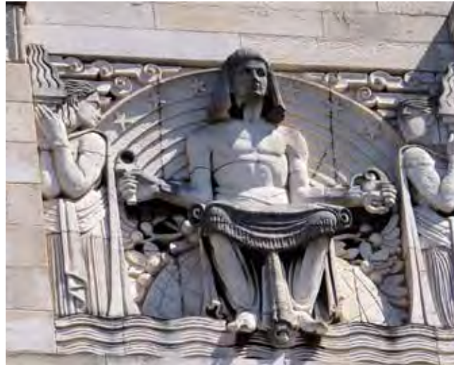
5. This fine building can be found on Surrey Street.
